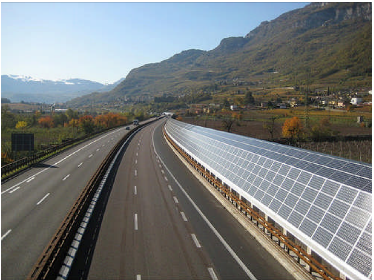
Figure 8: An example of a multifunctional integrated solution where photovoltaic cells are integrated into noise barriers.
